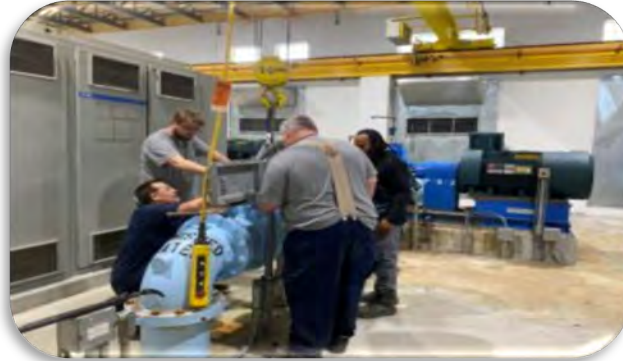
HIGH SERVICE PUMP REPAIR
